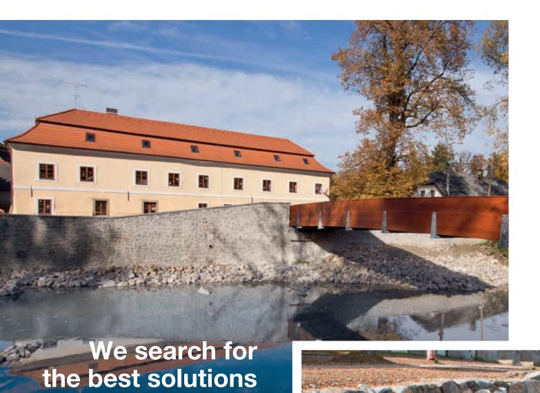
Residents of the town of Vlašim have a new footbridge over the Blanice River. The original footbridge was flooded several times and eventually it was pulled down by the flood. The lower edge of the footbridge structure is designed 0.5 m over the one-hundred-year flood level.
