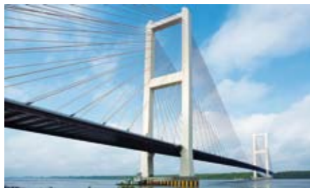
John James Audubon Bridge, USA
